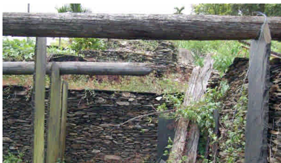
照3-7：舊筏灣家屋內石板柱與木梁 50
